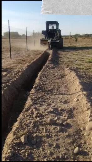
RT Barrera gets water system installed
